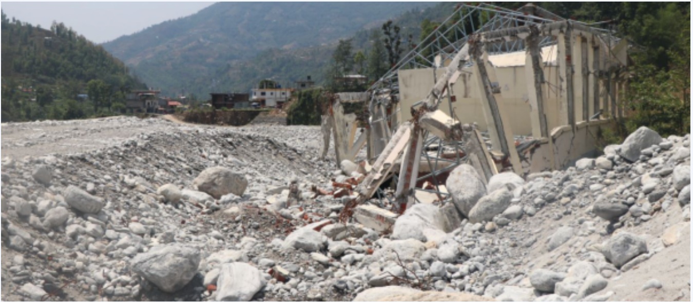
Aftermath of the flood and debris flow in Melamchi in June 2021, (Image: Yutshu Shrestha)
